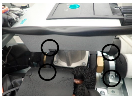
Fig8. Removing clamps
