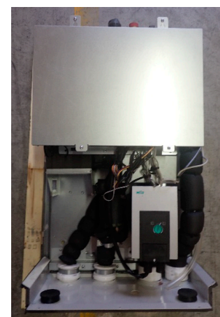
Fig4. HMU with cover removed
