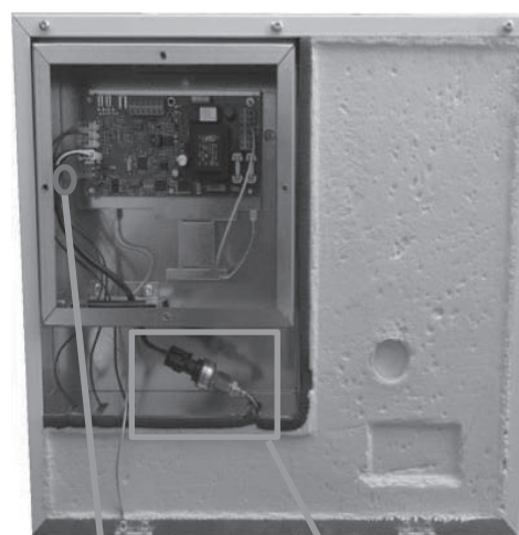
BP4 connector Pressure sensor (BP4)
