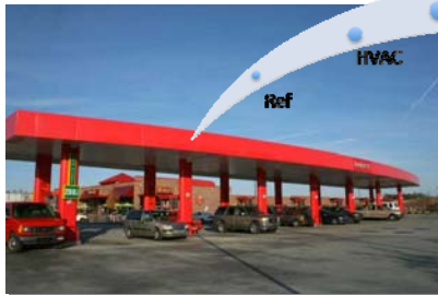
Sheetz C Store, Baltimore, USA
